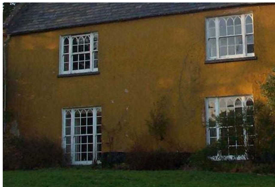
8 Vertical sliding sash with Gothic detail
